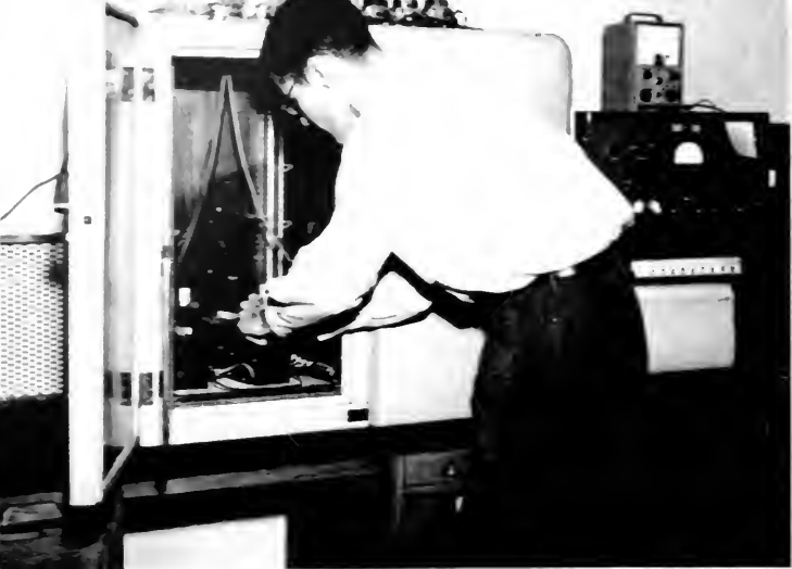
Measurement of Bacterial Growth by Constant Rate Nephelometer Dairy Research Laboratory
